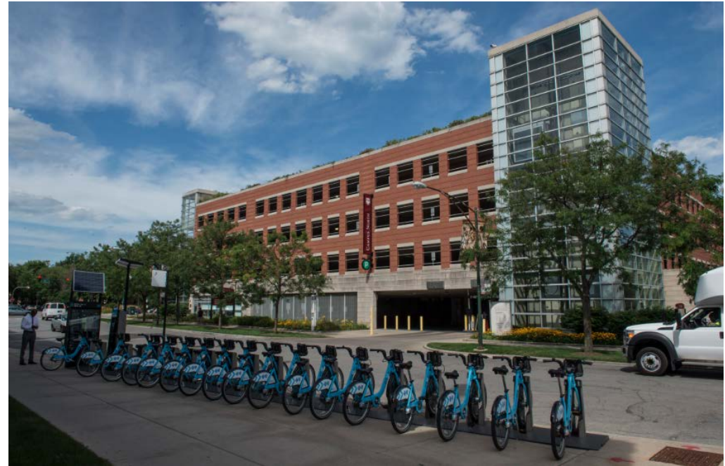
University of Chicago Parking Garage
