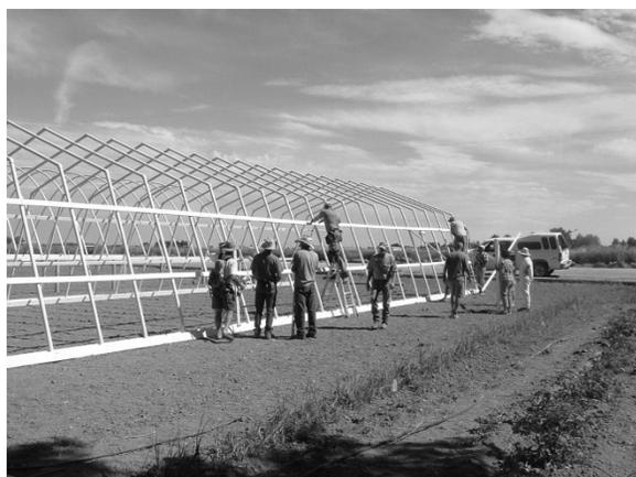
**Figure 3.** High tunnel construction (the Gothic type).
