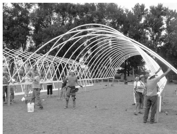
**Figure 4.** High tunnel construction (the two-sided type).
